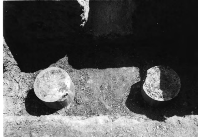
Large concrete piles as part of the foundations selected due to the nature of the terrain.
