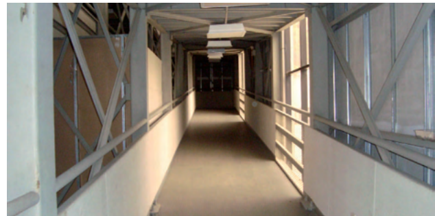
Interior of the external ramp.
