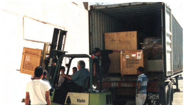
As the doors of the building were not wide enough to admit the bulky boxes containing the equipment and accessories, it was necessary to use a forklift to lift and lower the equipment from the outside.
