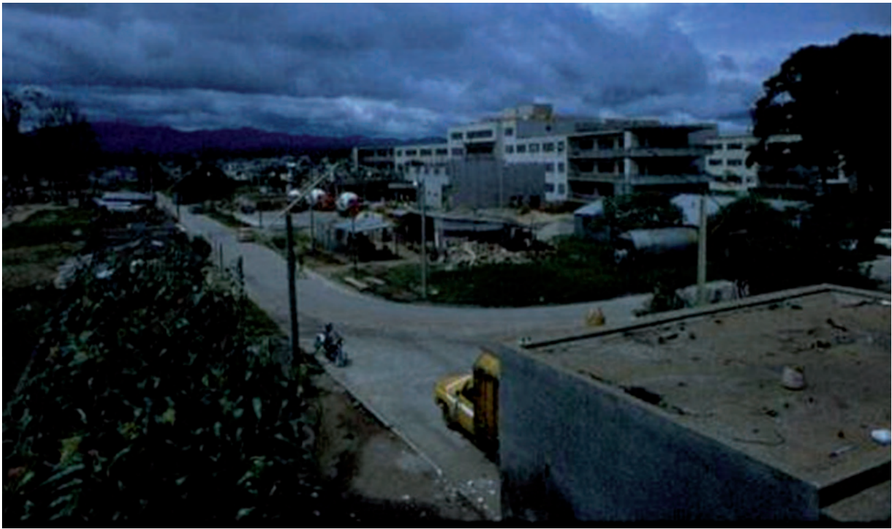
The large 4-level building corresponds to the back part of Roosevelt Hospital. In the front part, the construction area of the UNIT can be seen.
