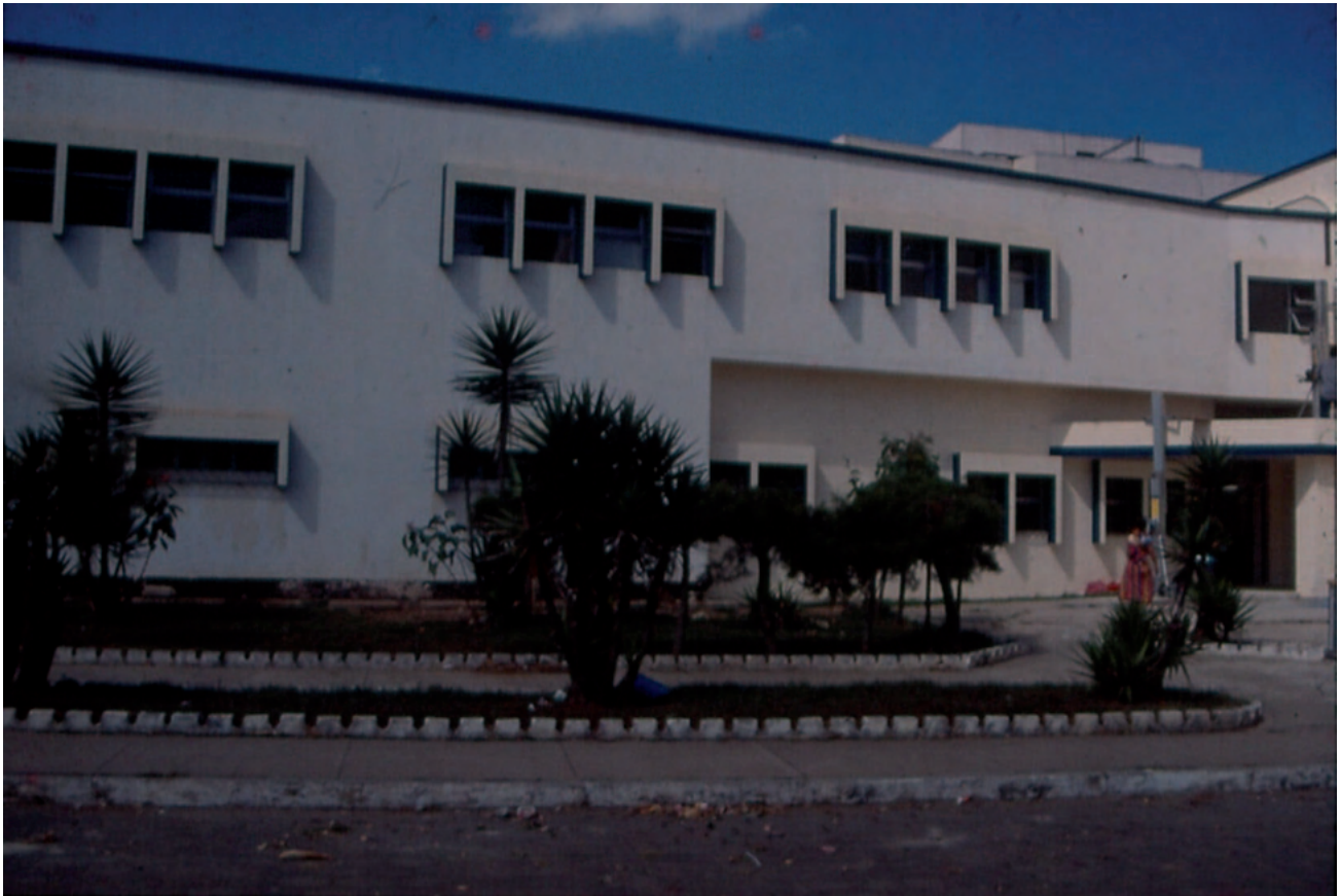
The building facade was finished and painted.
