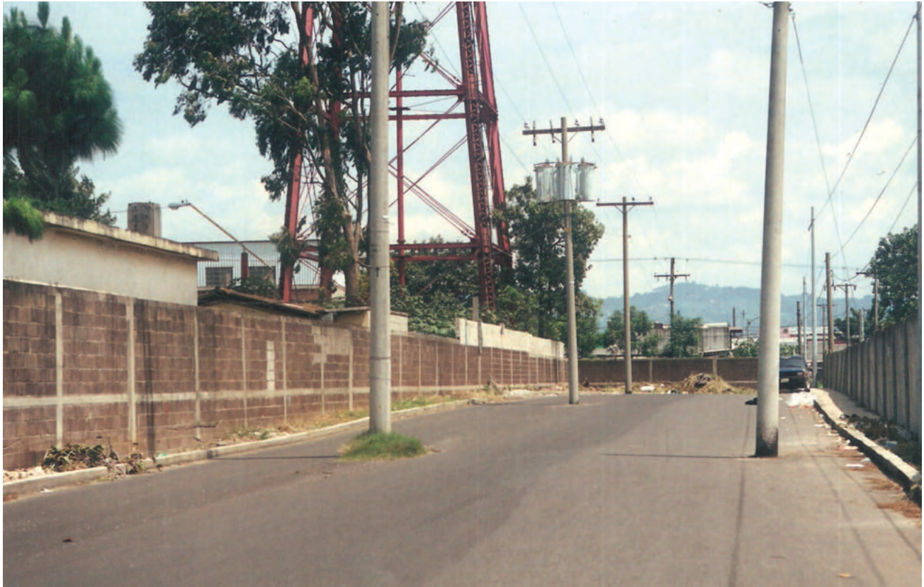
Street of Poles properly asphalted.
