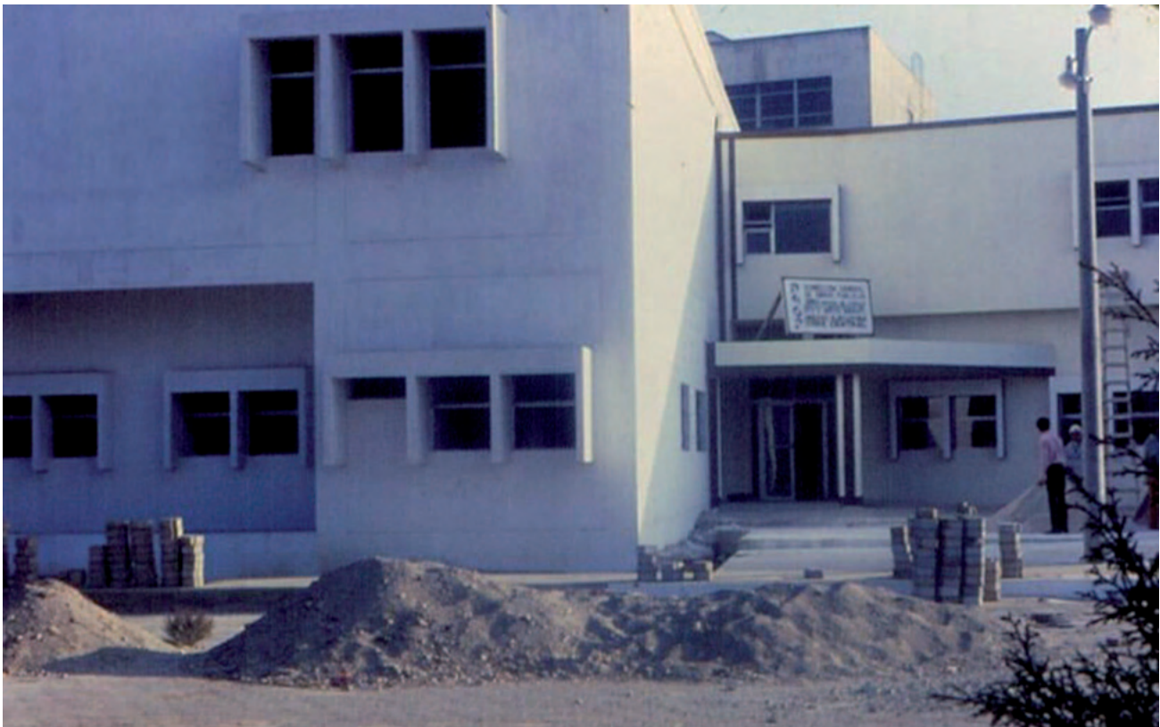
The front view of the Cardiovascular Surgery Unit under construction.
